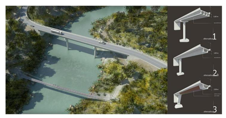
It is a bridge over the Torola river with 4 spans of 32.5m each in a high seismicity area. The 9m wide deck is composite and is composed of 4 steel beams of 1.10 m height and a top slab of 0.25 m concrete.
